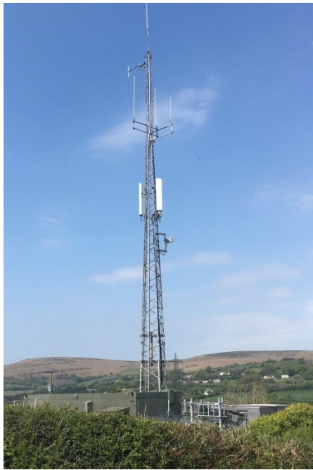
'BT TELECOM TOWER'
